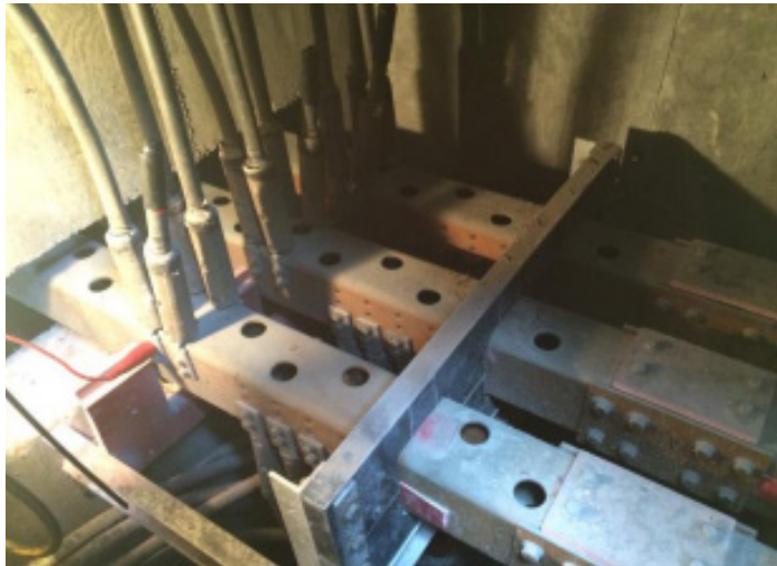
Previous Exposed Bus Configuration
