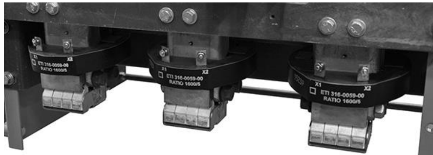
Figure 10: Lower Network Protector Contacts
