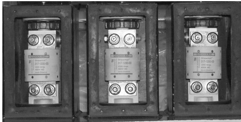
Figure 9: External Fuses
